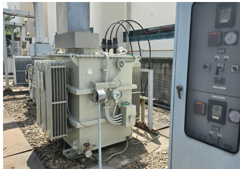
After Replacement (Hybrid Transformer)
