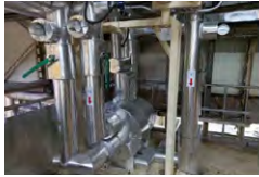
Photo of high-efficiency heat exchangers installed
