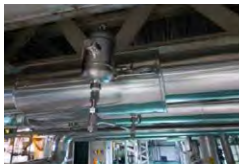
Photo of steam flowmeters installed
